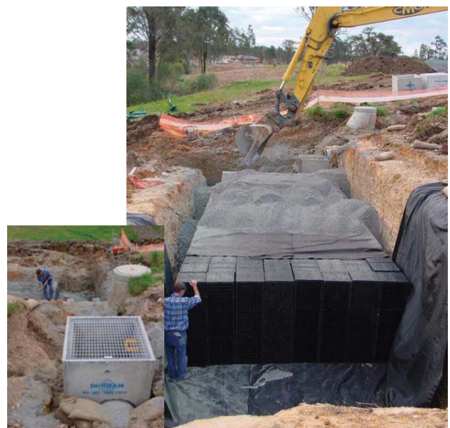
VersiTank® Infiltration System being installed
