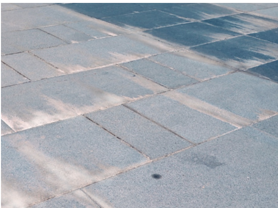
Efflorescence manifests as unsightly white patches on tile surfaces
