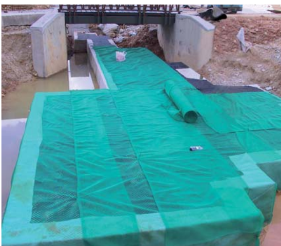
VersiTank® Infiltration System and the completed 'Rain Garden'
