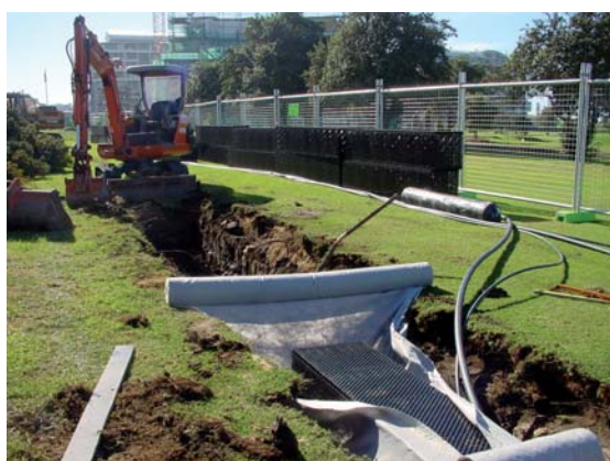
VersiTank® Infiltration System used in a trench application
