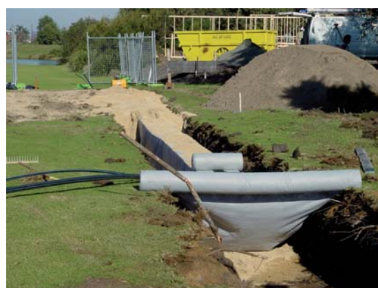
VersiTank® Infiltration System used in a trench application
