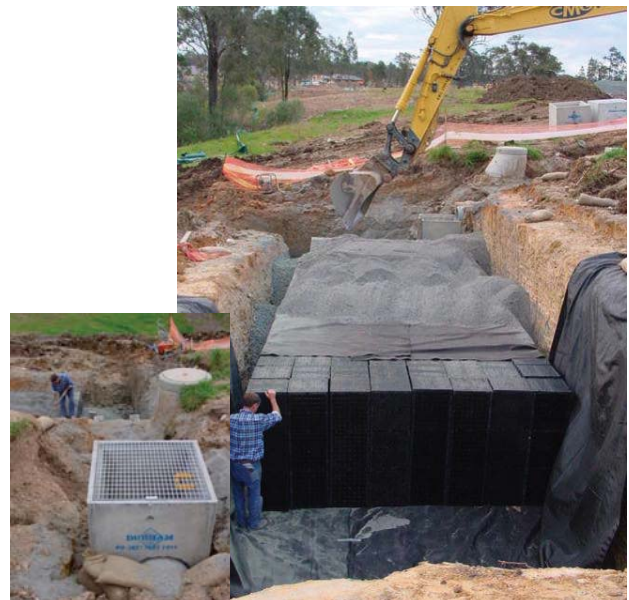
VersiTank® Infiltration System being installed
