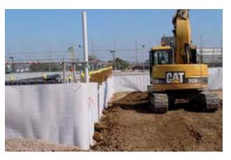
VersiDrain 8 Geo provides efficient drainage of basement and retaining walls and waterproof membrane protection
