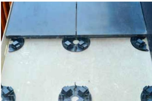
VersiPave® separated into halves to enable flush placement along edges.
